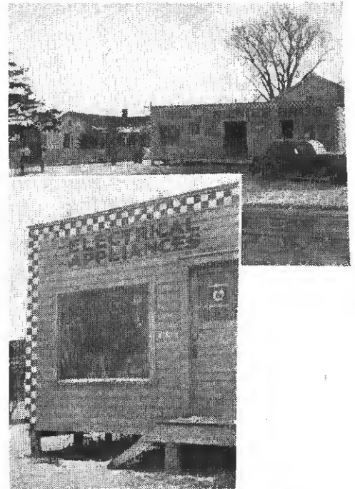
WEST ALLIS, Wis. —Riemer Bros., 9633 W. Greenfield Ave., feed store and electrical appliance shop. Been selling radios and appliances for past 10 years. Last year that appliances were available they sold 175 radios, 135 refrigerators; over 100 washers. Now specializing in service.
